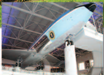
The cogeneration system at this prestigious presidential library and Air Force One Pavilion in Simi Valley, California, generates 960 kW of electric power, and the microturbine exhaust drives absorption chillers that provide 387 tons of air-conditioning.
