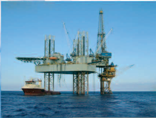
This unmanned platform relies on four C65 Capstone MicroTurbines to produce its continuous power needs.
